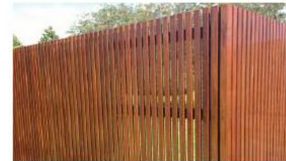
6. Timber slatted external plant enclosure
